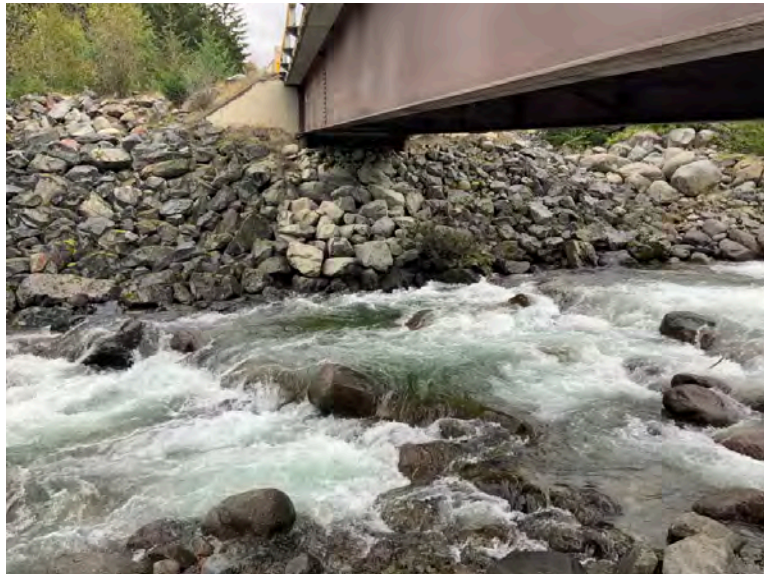
Right Bank Abutment when facing downstream
