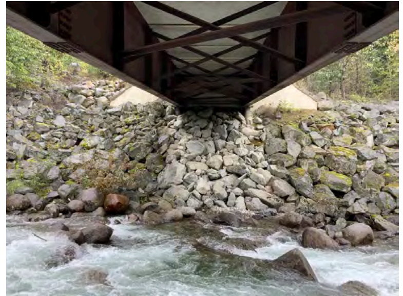
Left Bank Abutment when facing downstream
